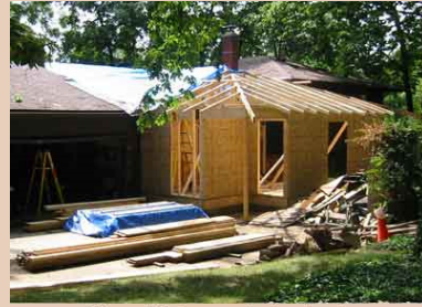
The addition to the back of the Goold Residence, 2003
